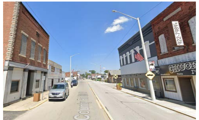
Figure 50: Boarded up upper floors in downtown buildings.
